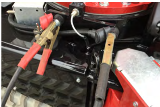
Figure 5.5 Bornes de recharge de secours
